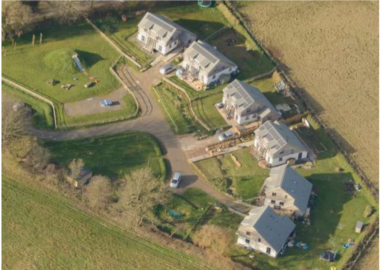
Broadhempston CLT – self-build
