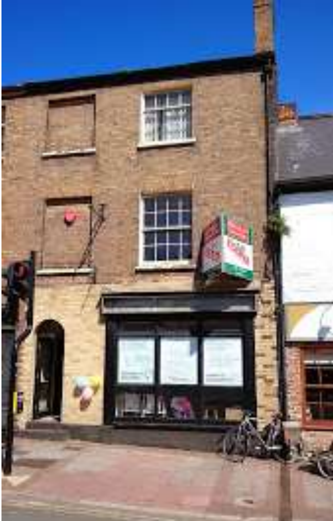
Somerset Co-operative CLT - refurbishment
